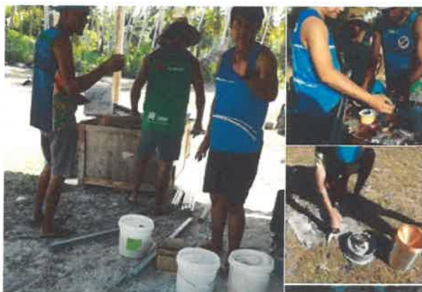
Figure 6 AWS installation in Cook Islands
